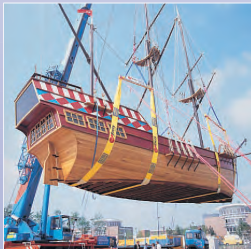
An 18 t. three-mast-ship is being lowered into the water by crane.
