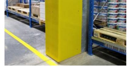
Collision protection for cement pile
